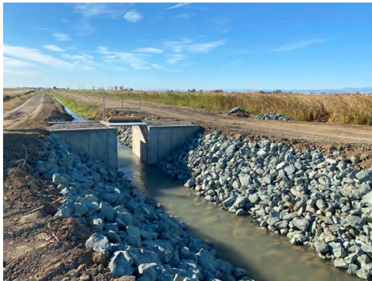
Figure 11. Existing Weir Structure on Lateral 16-4f
