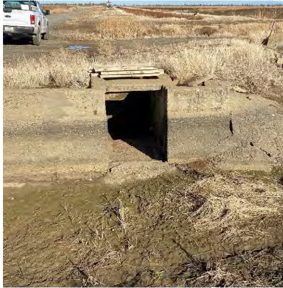
Figure 12. Existing Spill Structure on Lateral 41-1.
