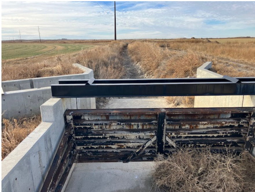
Figure 2. Current diversion works at Lateral C.
