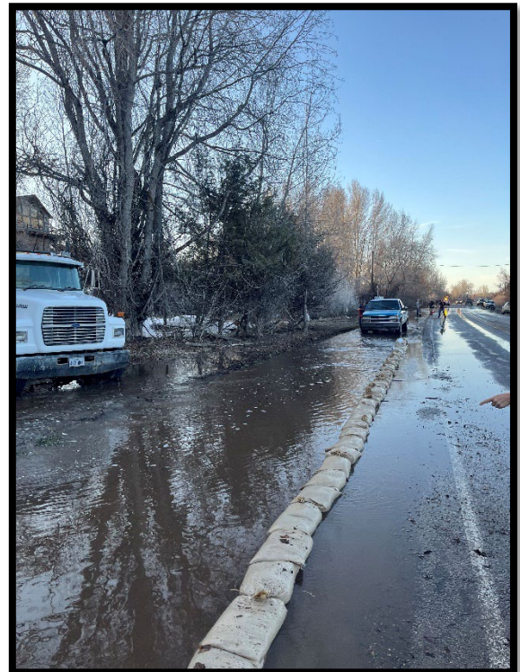
Photo 6 Flooding on the roads in Garden City Spring 2023
