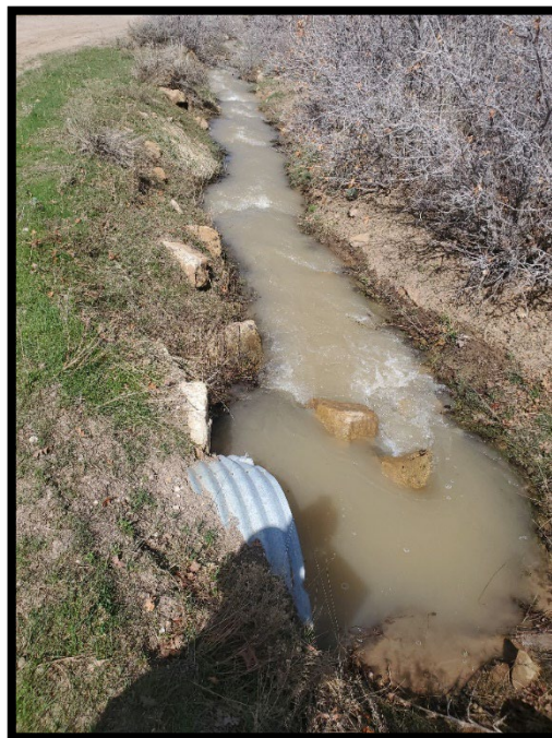
Photo 1 Earthen and old unlined ditches
