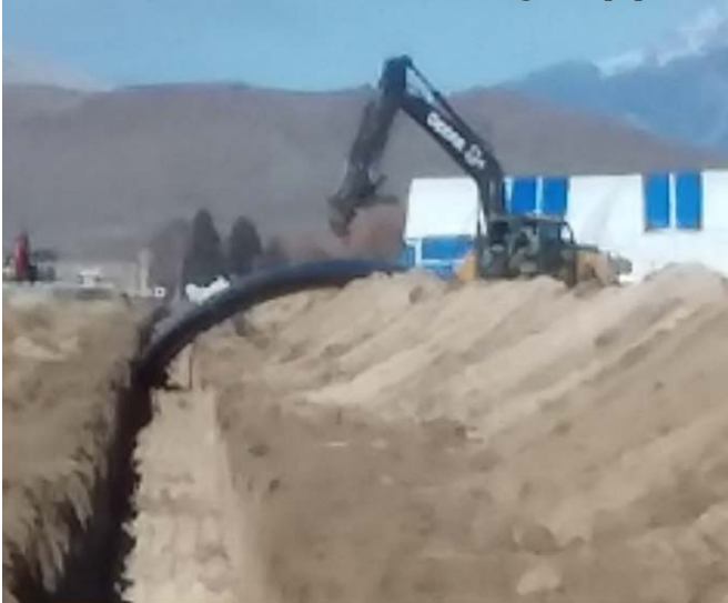
Picture 3 and 4: Phase 1 - Installing 30" pipe in Aikele Stubb Lateral
