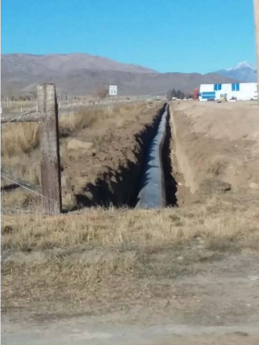
Picture 3 and 4: Phase 1 - Installing 30" pipe in Aikele Stubb Lateral
