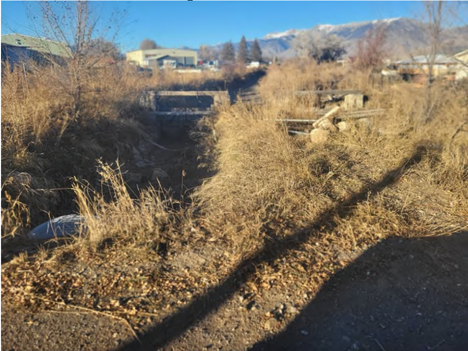
Picture 2: Phase 2 – Existing Westside Lateral
