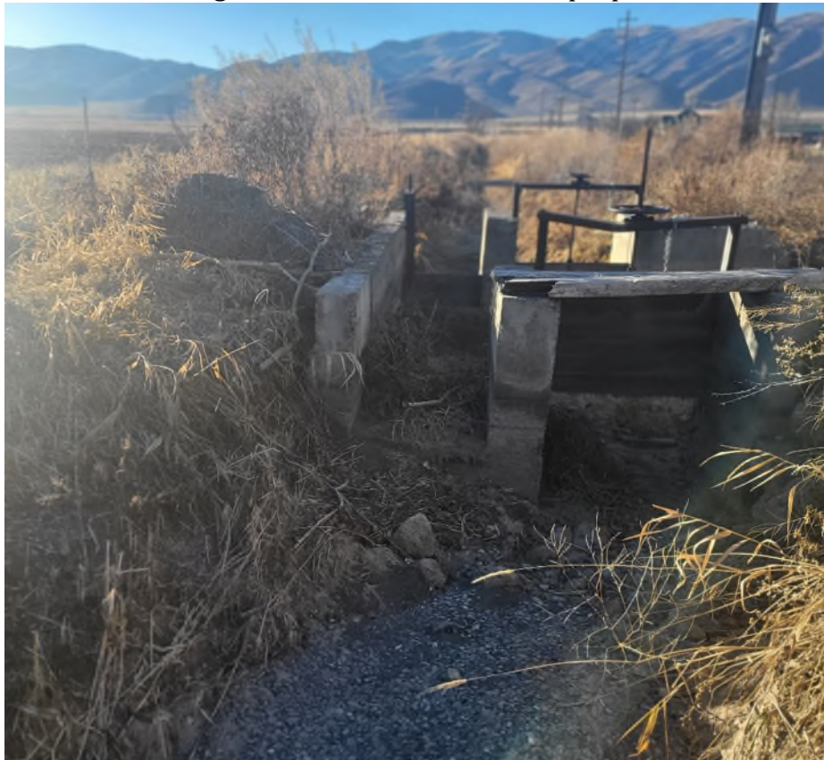
Picture 1: Existing Canal and infrastructure in proposed Phase 2 location
