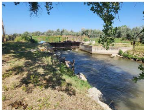
EXISTING CONCRETE HEADGATE STRUCTURE - DOWNSTREAM
