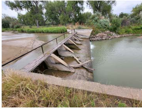
EXISTING CONCRETE DIVERSION STRUCTURE - DOWNSTREAM
