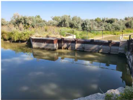
EXISTING CONCRETE WASTEWAY STRUCTURE - UPSTREAM
