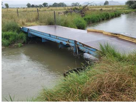
EXISTING STEEL BRIDGE
