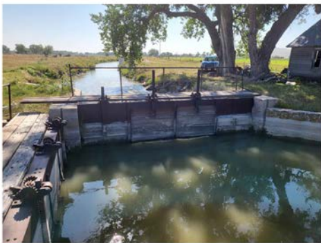
EXISTING CONCRETE HEADGATE STRUCTURE - UPSTREAM
