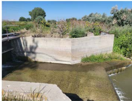
EXISTING CONCRETE WASTEWAY STRUCTURE - DOWNSTREAM
