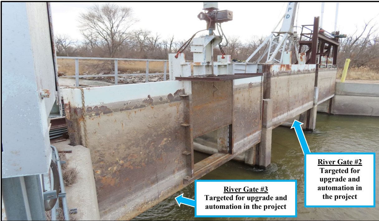
Figure 5. Dawson County Canal River Gates 3, 2, and 1 (from left to right)
