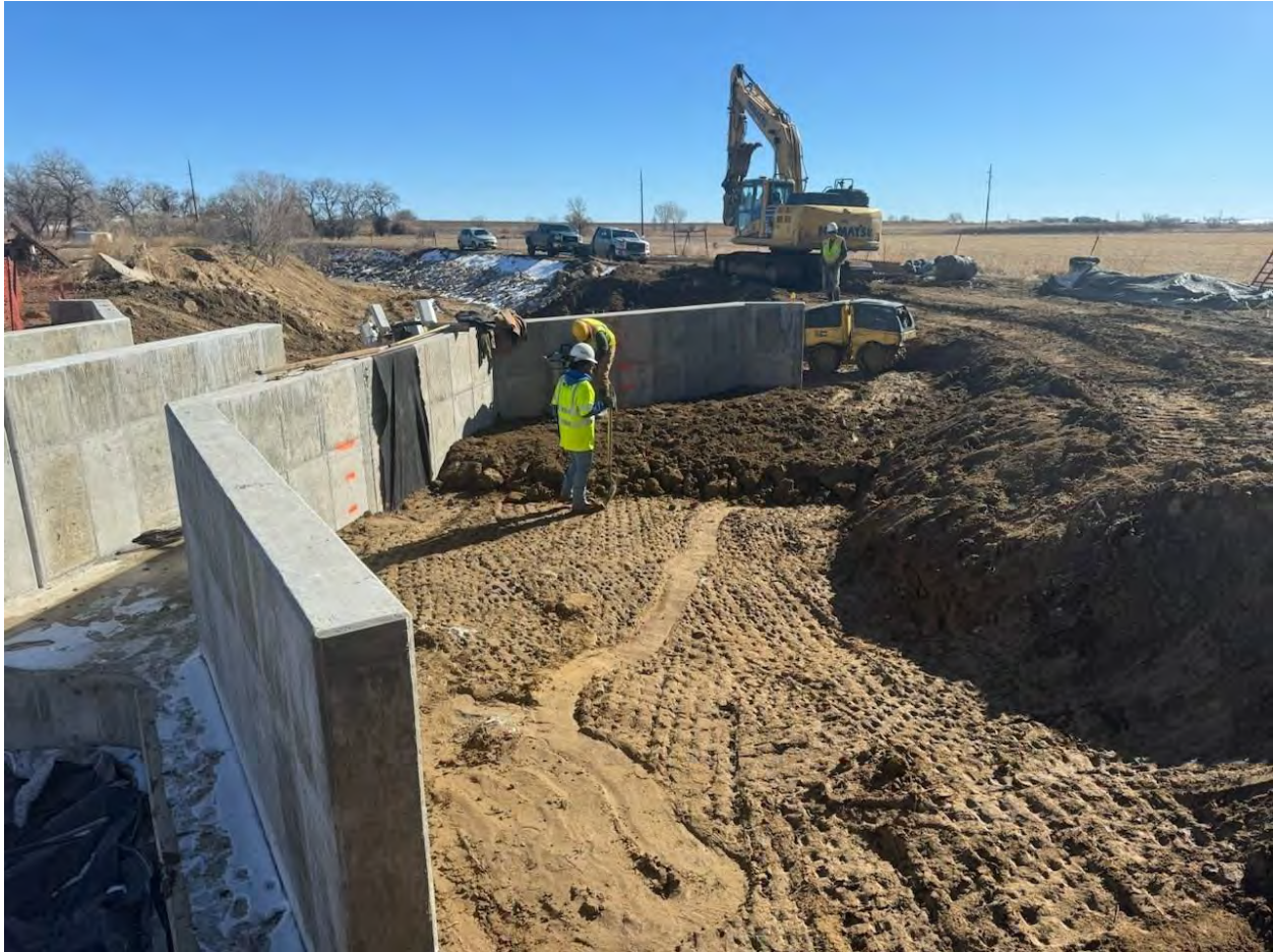
Figure 3. 2023 Single Flumegate Installation with Concrete Work Complete and Backfill Commencing
