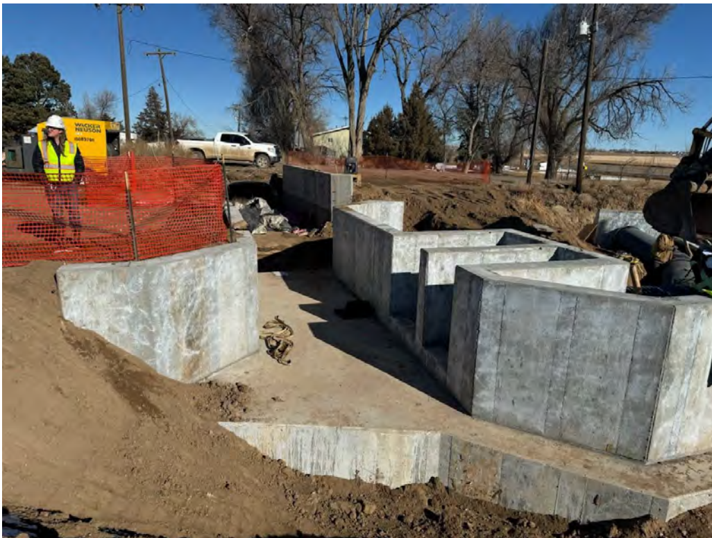
Figure 2. 2023 Double FlumeGate Installation with Concrete Work Complete and Backfill Commencing
