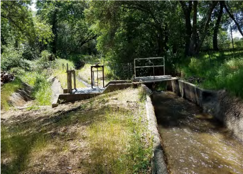
Figure 8. Before FlumeGate Installation
