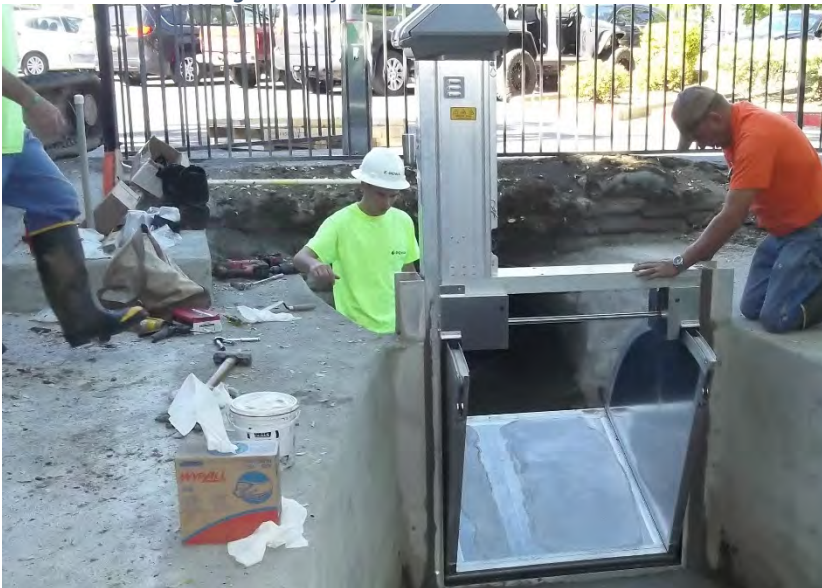
Figure 10. During FlumeGate Installation
