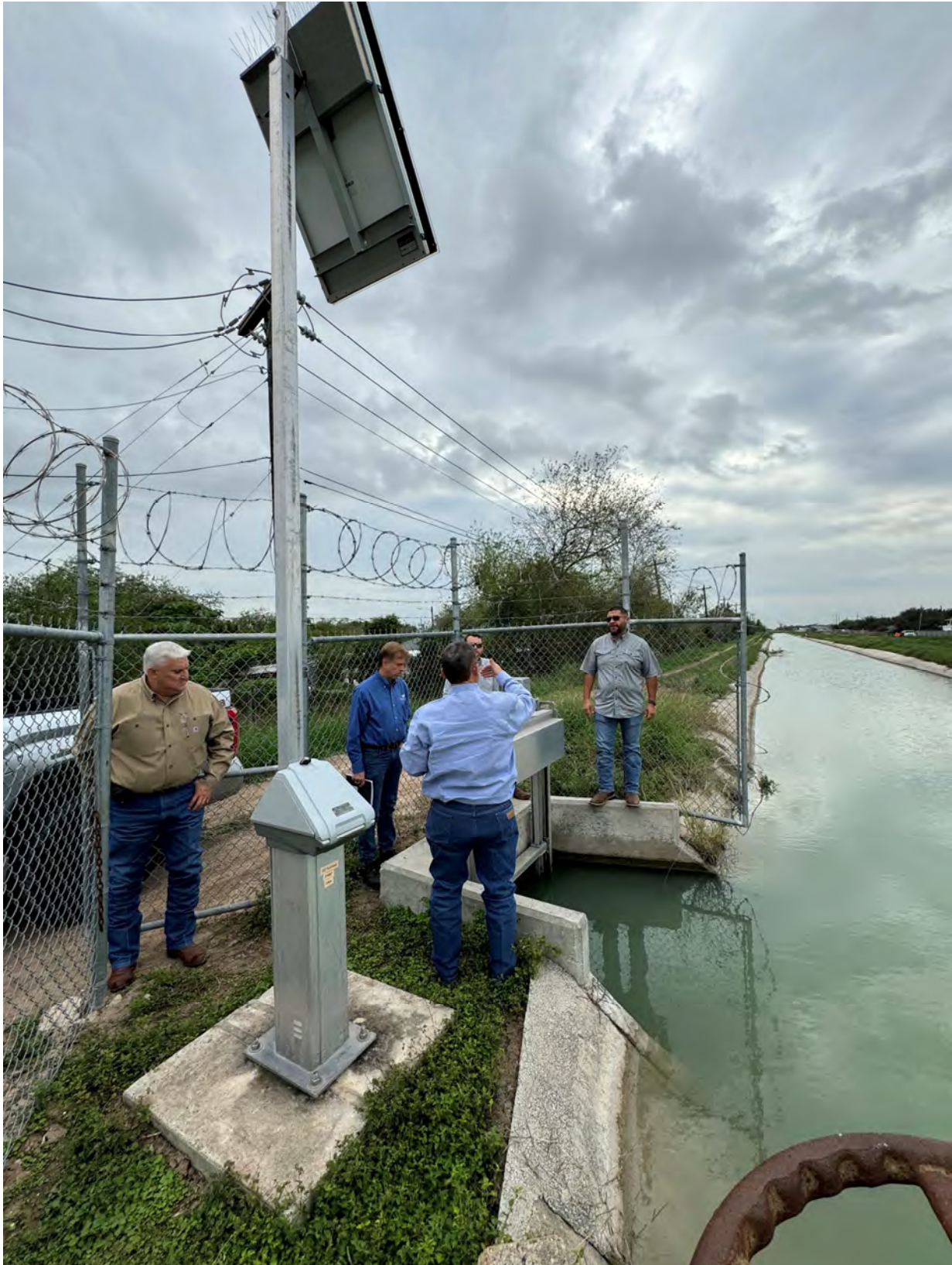
Figure 15 – Flow Control & Metering Gate with Solar Pedestal
