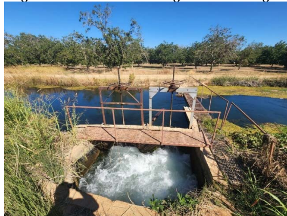
Figure 11. West Ditch existing headwall and gate
