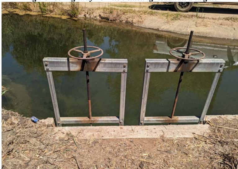
Figure 13. Highway 20 Ditch existing headwall and gate
