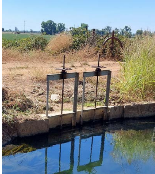
Figure 3. Example of existing sluice gates (Highway 20 Ditch)
