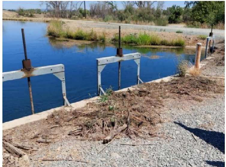
Figure 7. North and South Diversions existing headwall and gates
