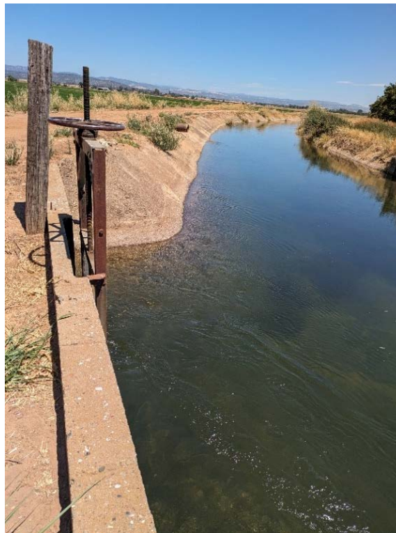
Figure 9. 7-Mile House Ditch existing headwall and gate
