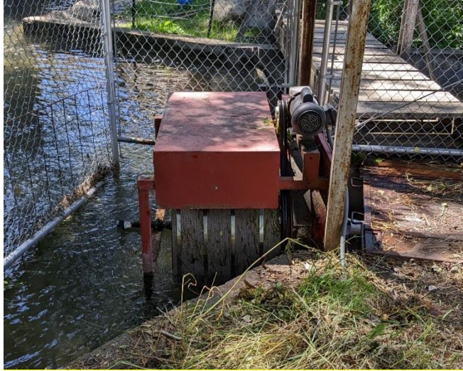
Figure 3: Three Creeks Diversion Structure
