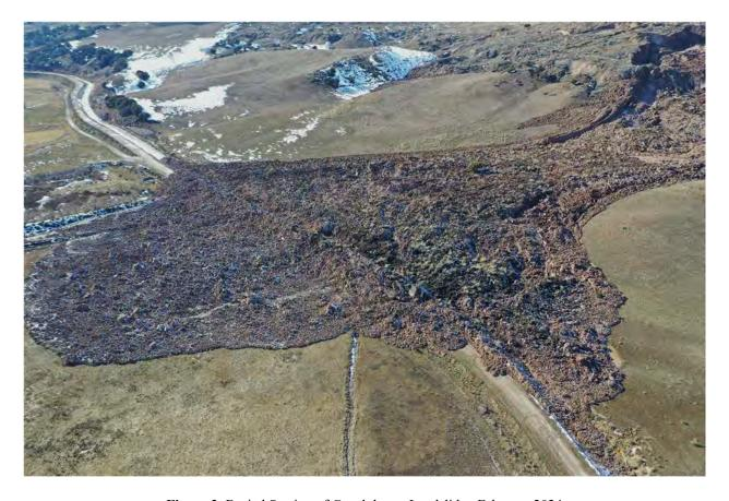
Figure 2. Buried Section of Canal due to Landslide-February 2024
