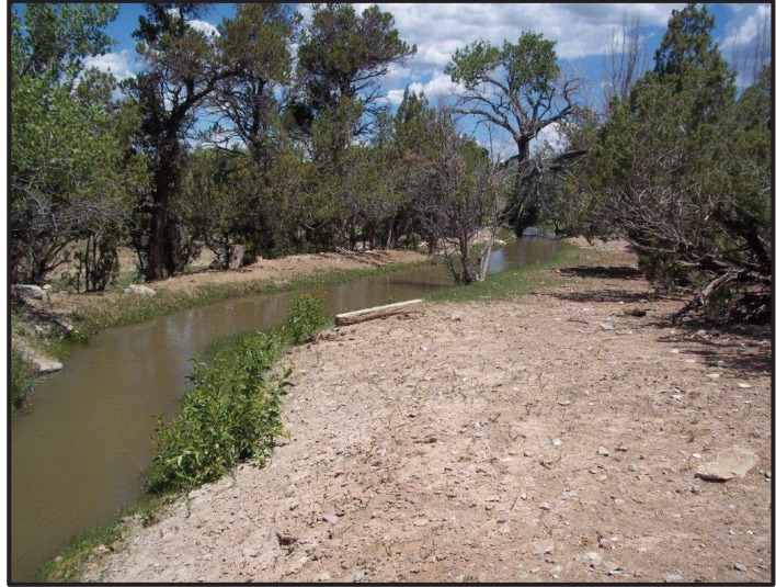
Photo 1: Water Loss Due to Evaporation and Seepage in the Lower Arickaree canal
