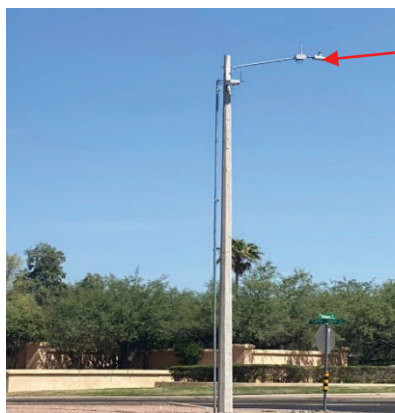
Itron CCU 100 and Repeater 100 have the same shape, size, and installation requirements
