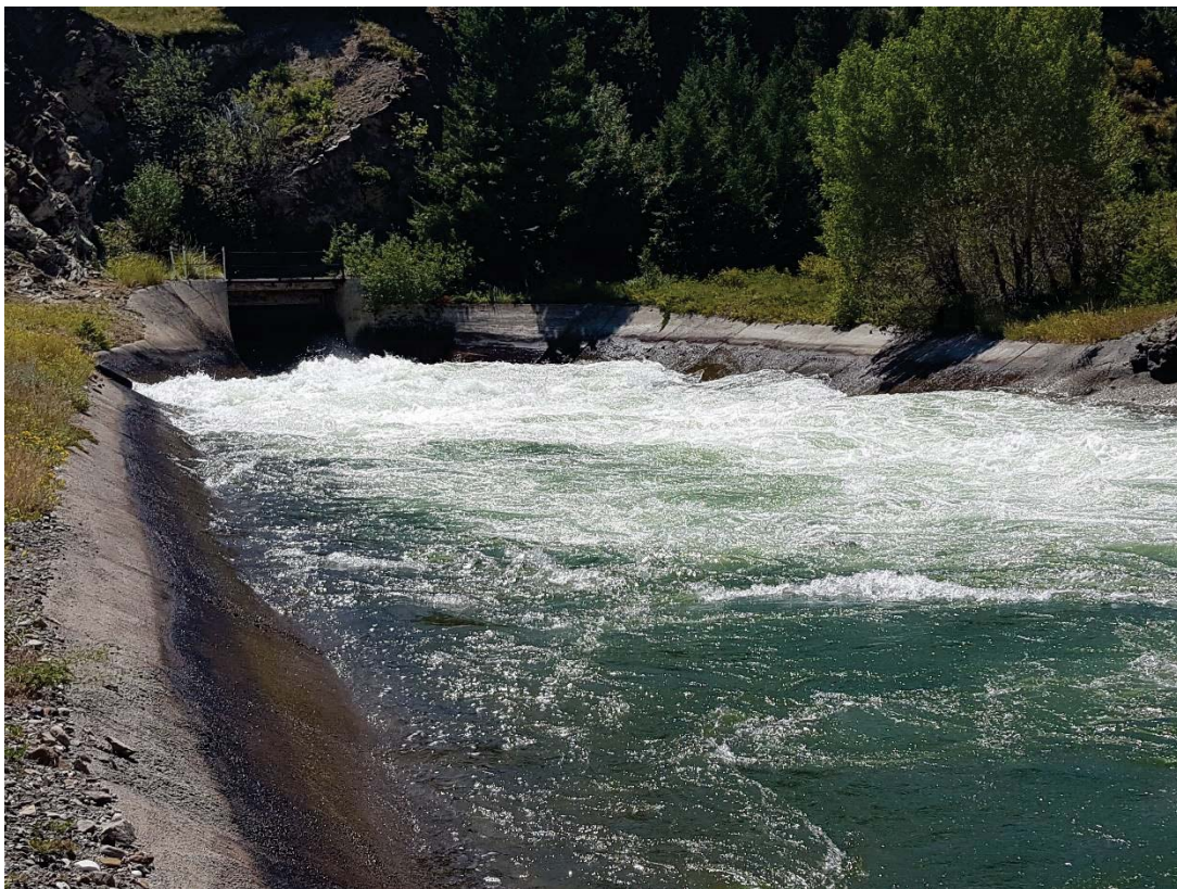
Photo showing outlet releases from Tunnel No.3, +/-1,350 cfs
