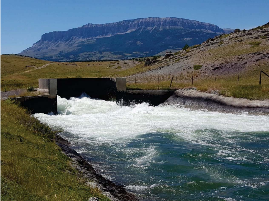
Photo showing outlet releases from Arnold Coulee Drop, +/-1,350 cfs
