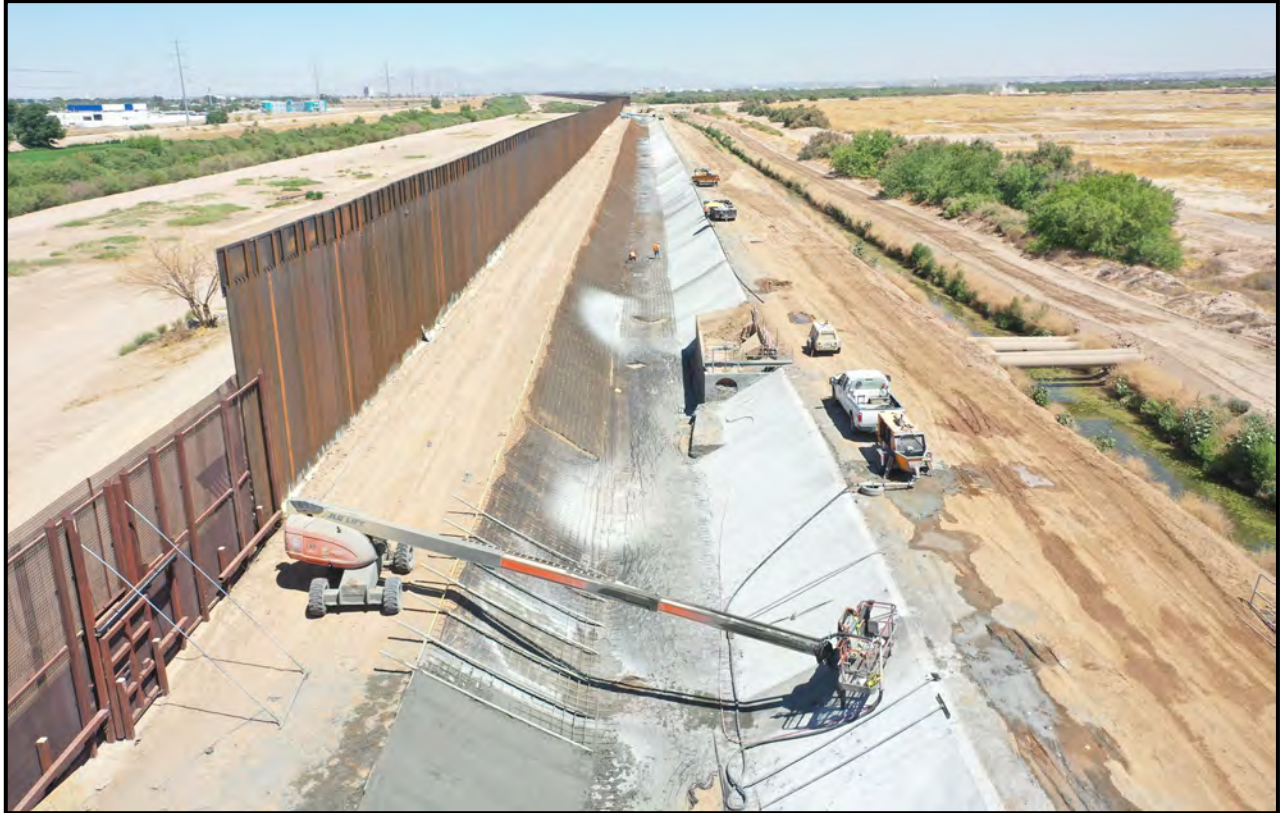
Figure 2. Phase II of Riverside Canal Concrete Lining Construction (2021)
