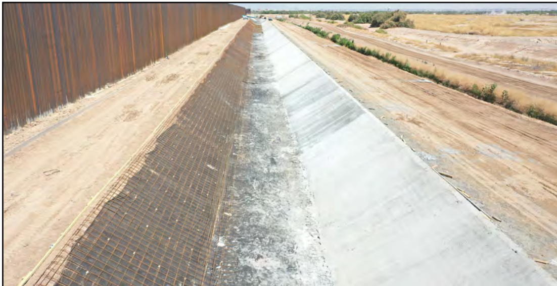
Figure 3. Shotcrete, Steel Panels, and Geofabric at Riverside Canal (2020)
