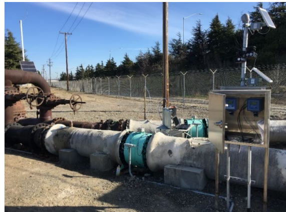
Figures 6 and 7 Examples of small and large AMI meter installations.
