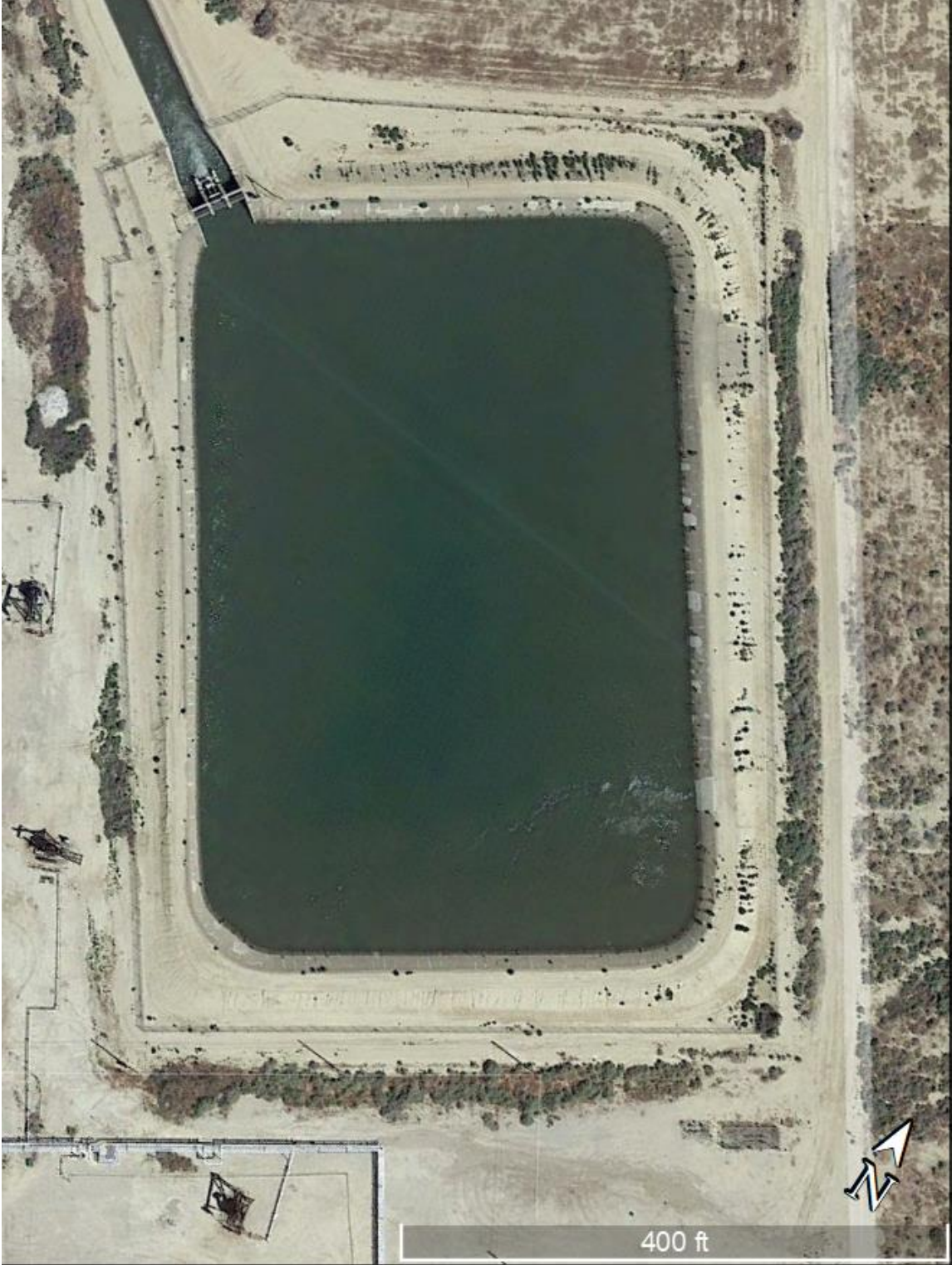
Photograph 2: Google Earth Aerial of 500 Reservoir
