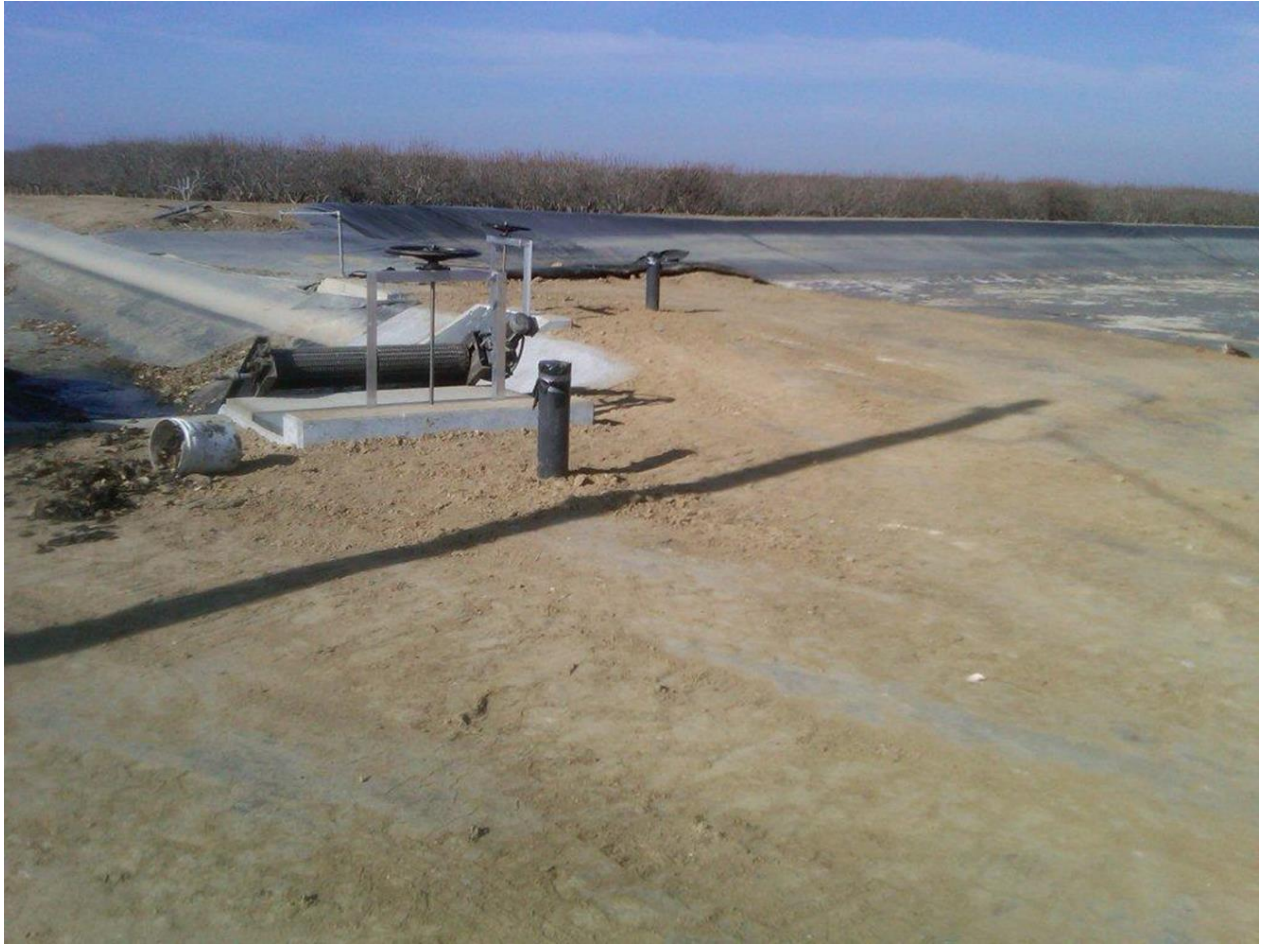
Photograph 3: LHWD SA-1 Reservoir 1-2 (has HDPE Liner, example of proposed liner in BWSD 415 and 500 Reservoirs
