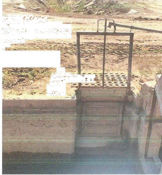
Photo 16 Kawai Lateral Head Gate/Turnout
