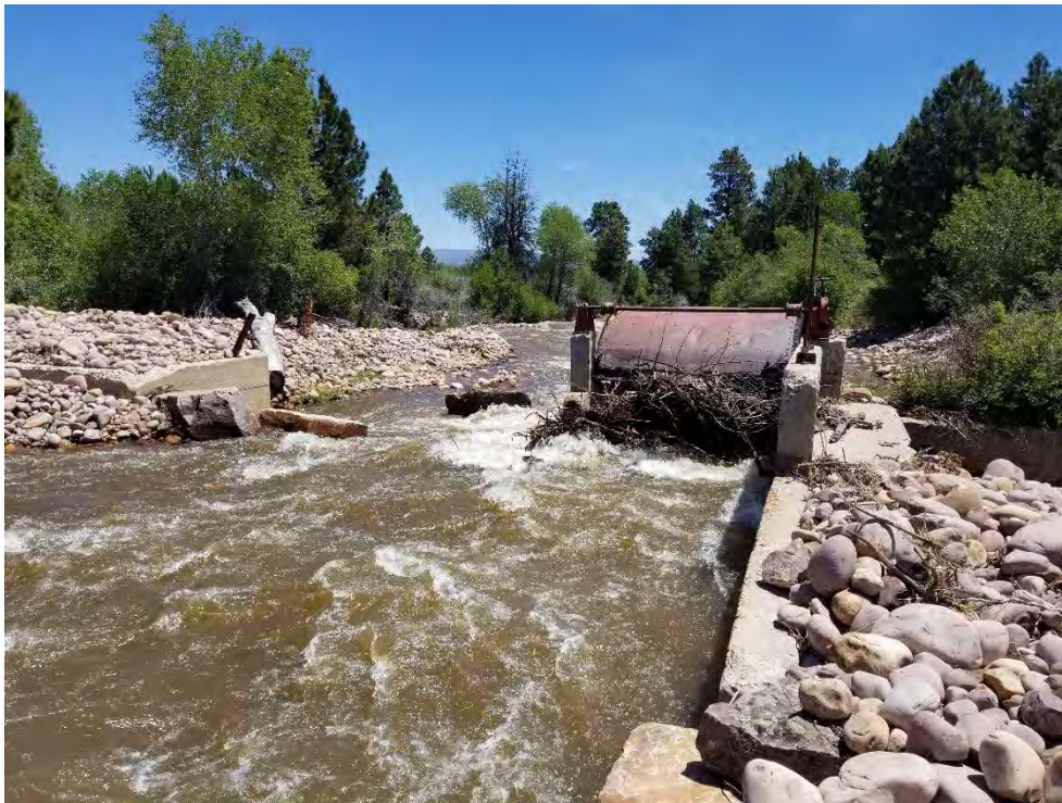
Figure 2: Existing Structure on Tribal Land
