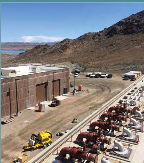
Low Lake Level Pumping Station Construction
