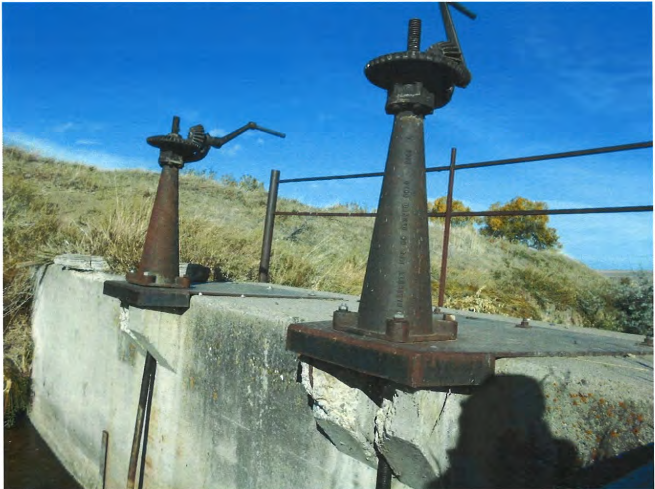
Inlet Canal Headgate
