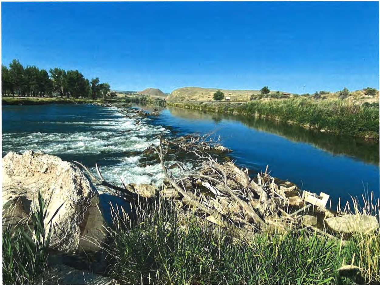
Diversion Dam on the Big Horn River
