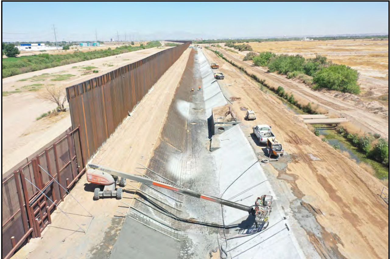
Figure 2. Riverside Canal Concrete Lining Construction (2021)
