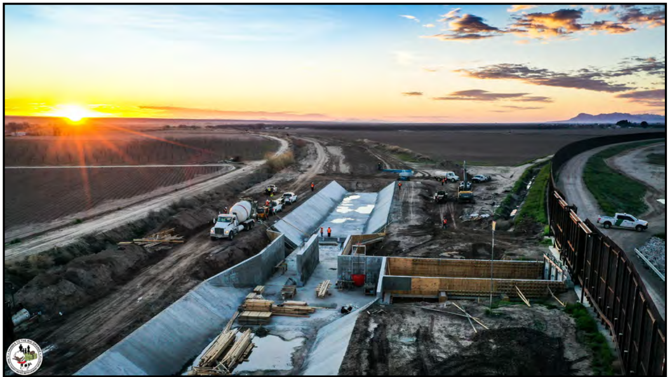
Figure 17. Reconstruction of Riverside Canal Wasteway II and Check Structures
