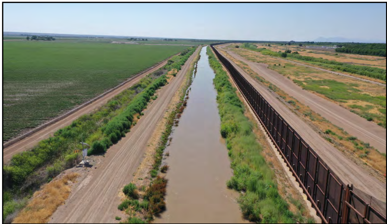
Figure 16. Typical Unlined Section of the Riverside Canal and Border Fence
