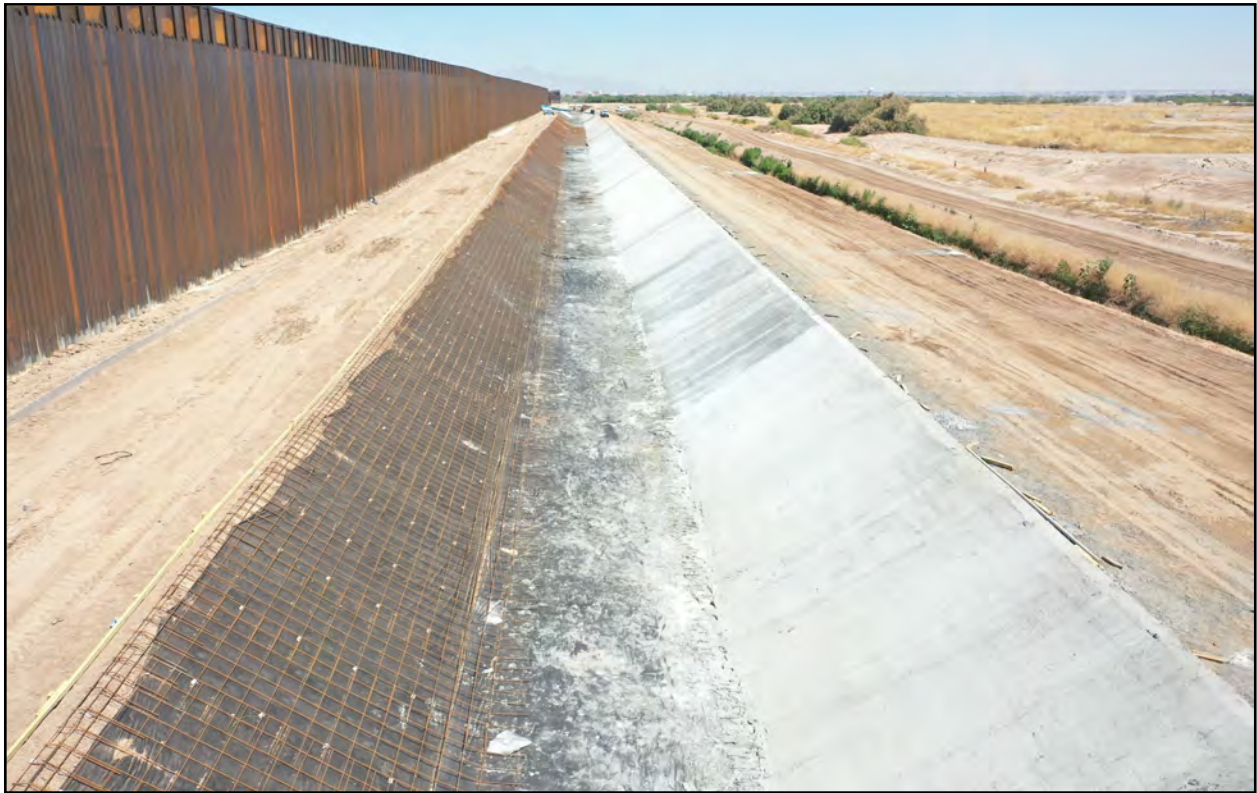
Figure 3. Riverside Canal Steel Panels and Lined Bank (2021)
