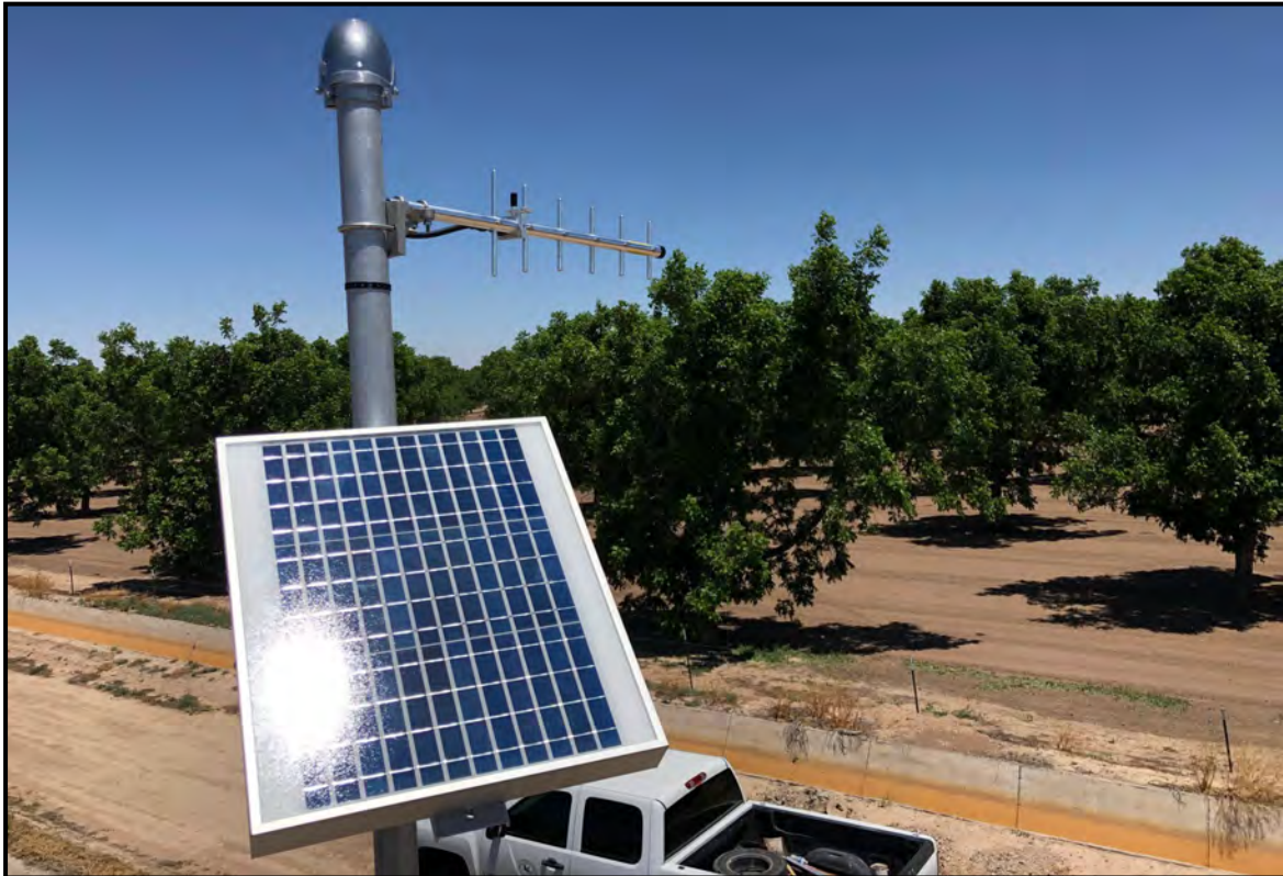
Figure 3. Solar Panel and Transmission Antenna at an EPCWID1 Lateral (2020)
