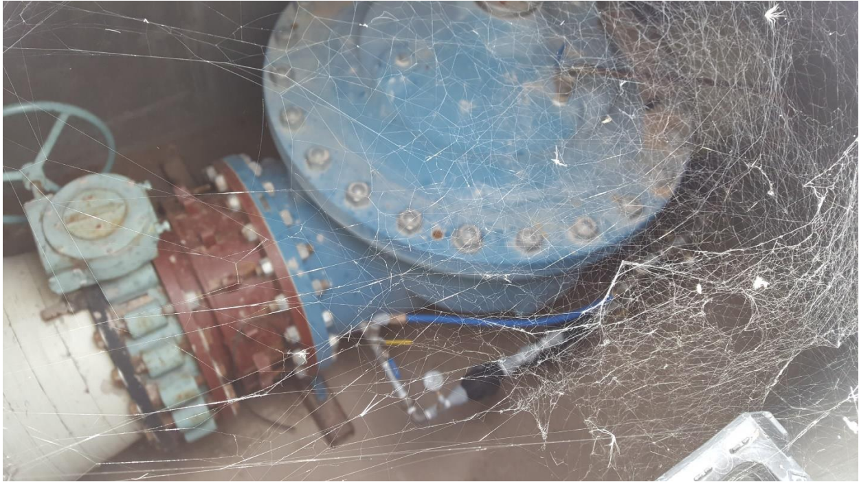
Figure 4: Goliath Pressure Sustaining Valve - To be converted to a PRV Upon Connection to Reservoir
