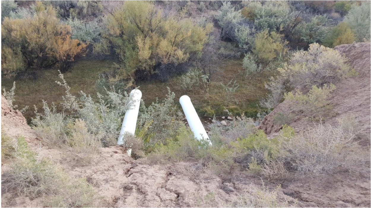
Figure 3: Cottonwood Spill Pipes Proposed to Be Abandoned by Closing System
