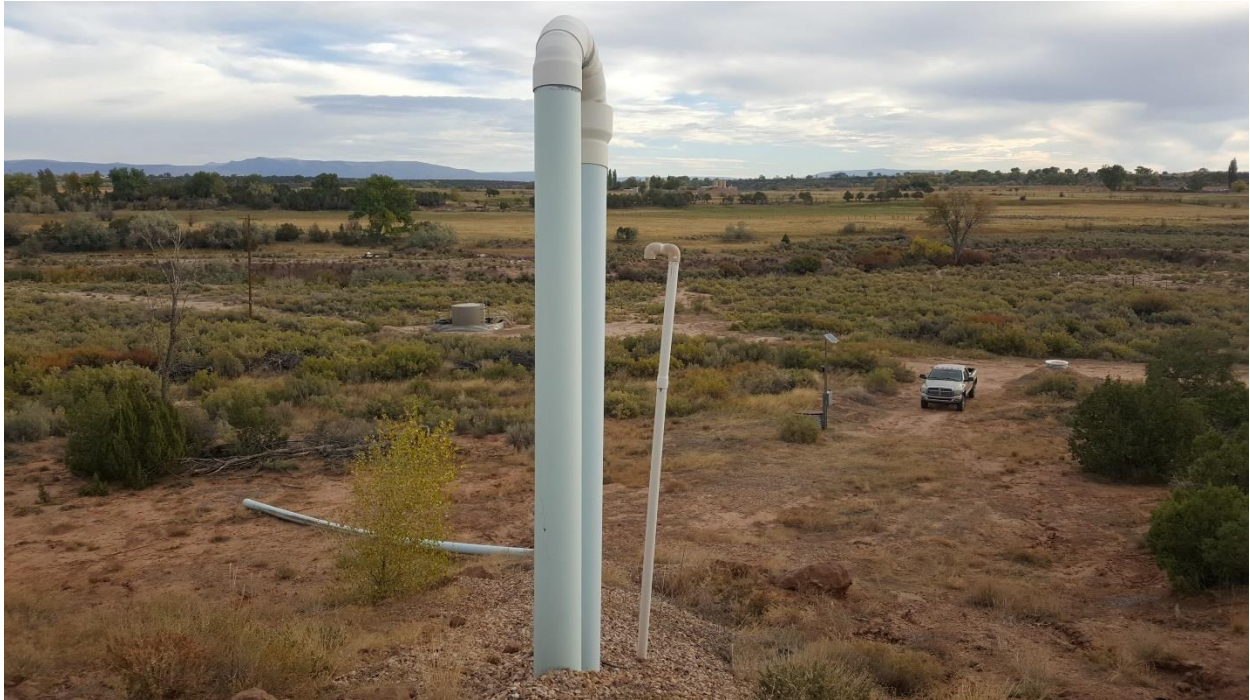
Figure 1: Cottonwood Spill Location and Stand Pipes
