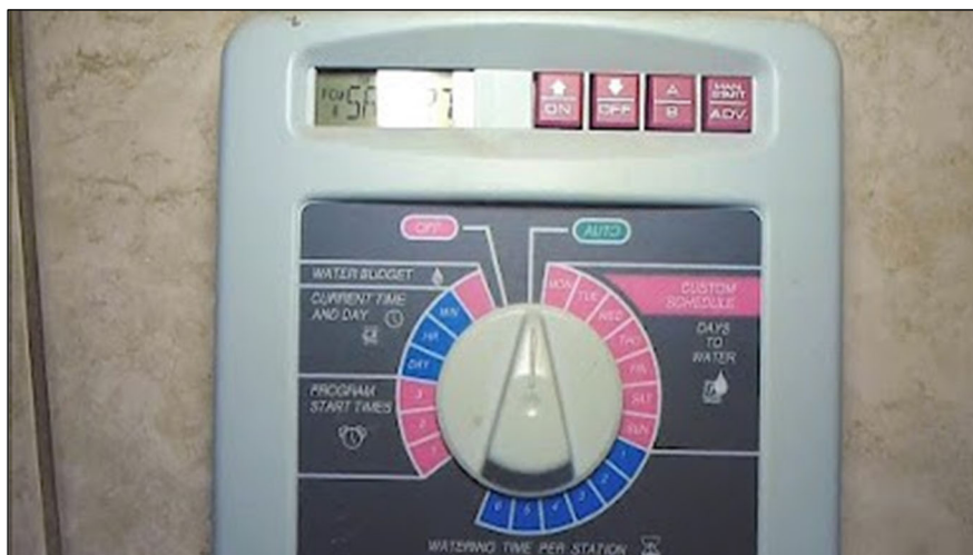
Source: City of Fresno DPU Staff Photo
