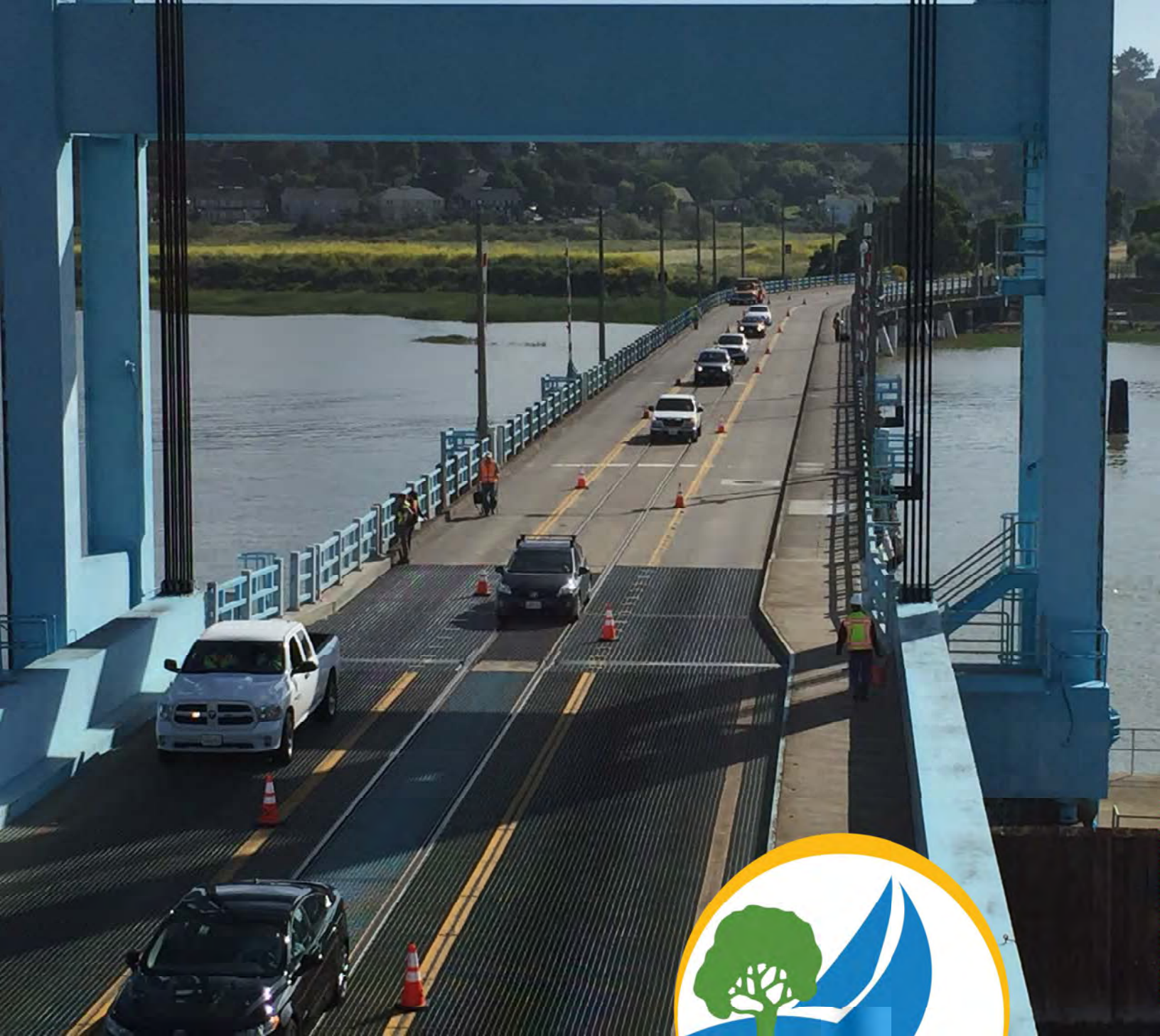
Mare Island Causeway Bridge
