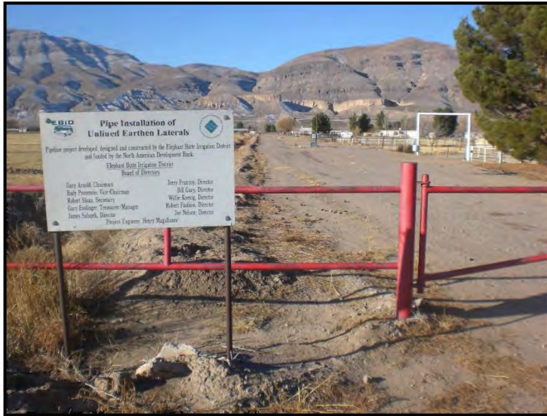
Figure 4: The Kerr Lateral, which has been placed in pipe.
