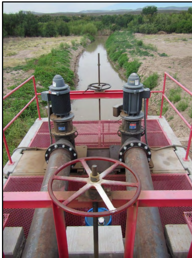
Figure 3. Pumps installed at the Rincon Wasteway 18
