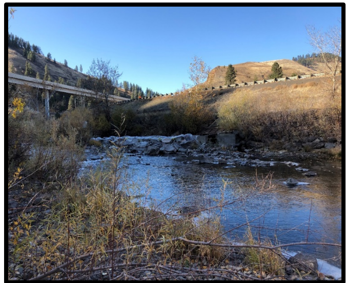
Figure 1 Grande Ronde River Near ICC Diversion
