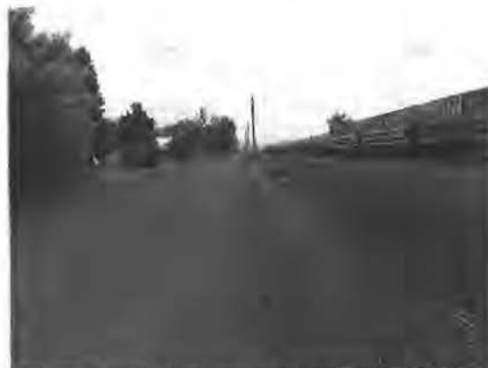
Harrison Avenue looking southeast down the Phase I pipe alignment.
