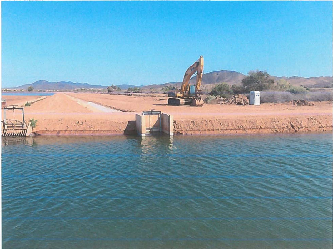
Figure 13: Completed Head Gate from Reservation Main to Acoma Lateral
