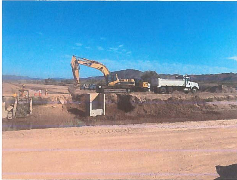
Figure 11: New Head Gate Installation for Acoma Lateral
