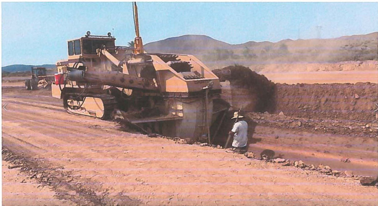
Figure 2: Trencher Creates Prism
