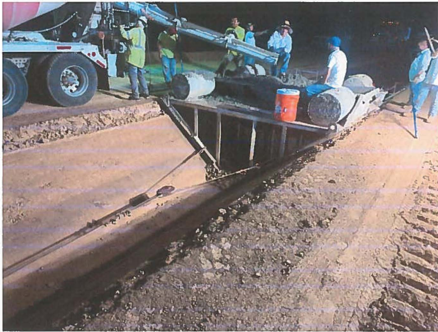
Figure 7: Concrete Poured In-Place for Gate
