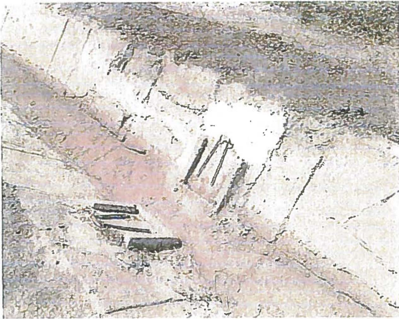
Image 3. Bard, CA. Example of distribution port in collapsed earthen embankment.
