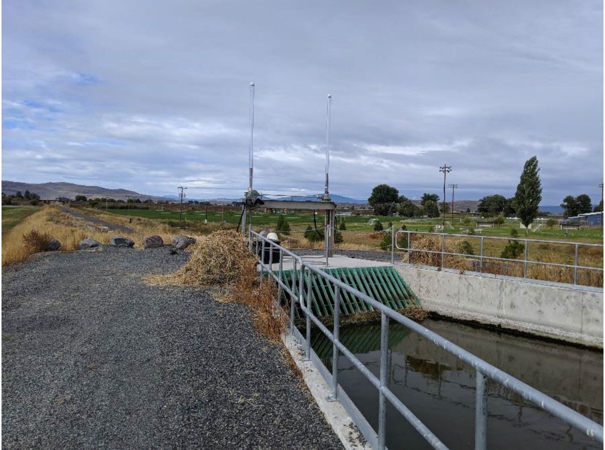
Figure 4 C-Siphon Gate with no automated controls. Flow inaccuracies are common due to human error and significant guesswork in flows upstream from the gate.
