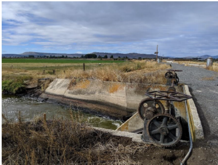
G Canal Gate
