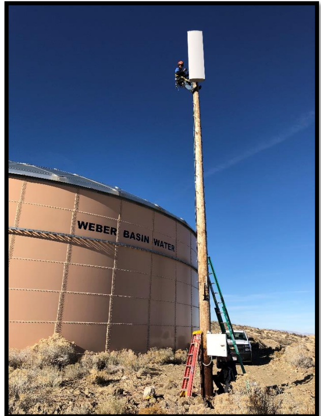
Photo 2 - Little Mountain Water Tank
