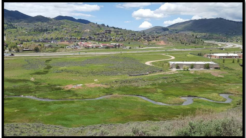
Photo 1 - East Canyon Water Treatment Plant
