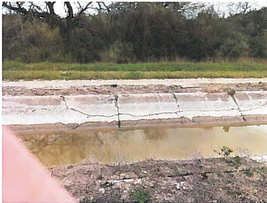
Picture 1. (Background) Visible horizontal crack in the east side slope. Horizontal cracks extend for the entire canal length on both interior side slopes.
