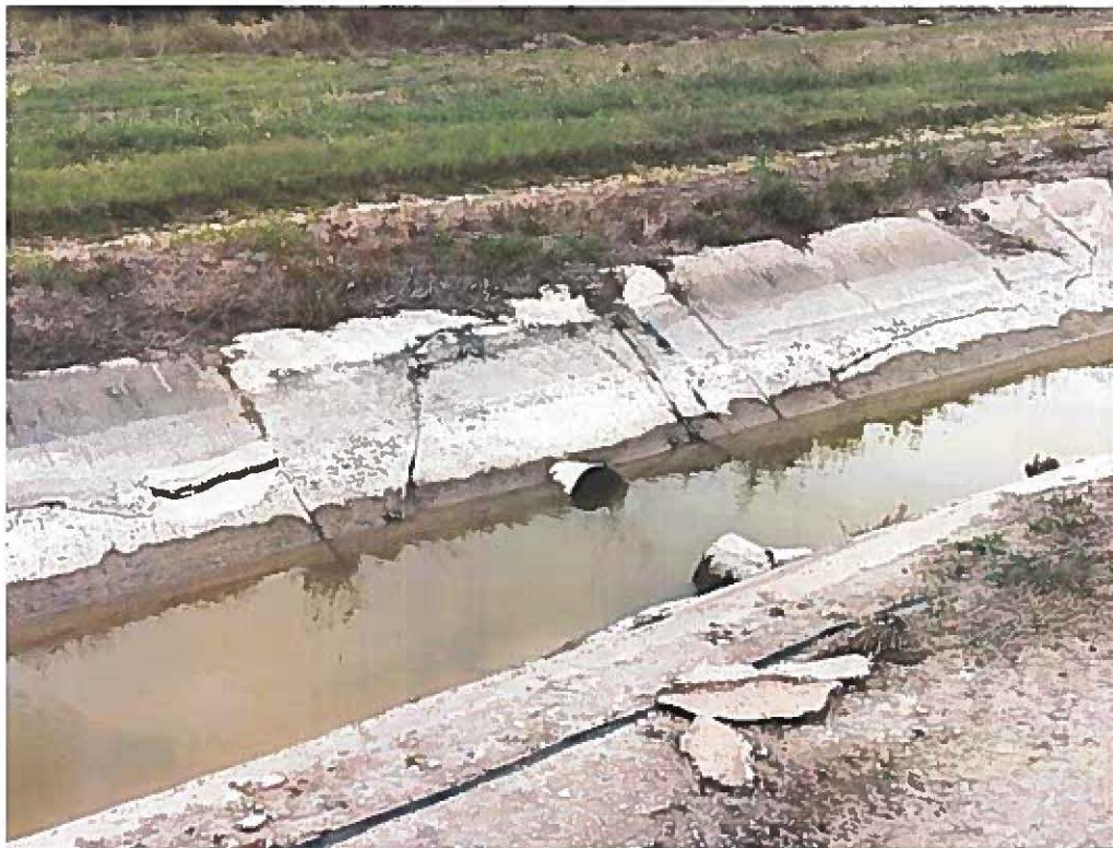
Picture 5. Typical field outlet pipe laterals.
