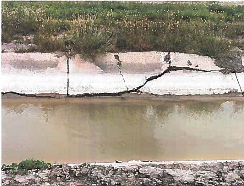
Picture 2 Visible buckling and structural movement.
