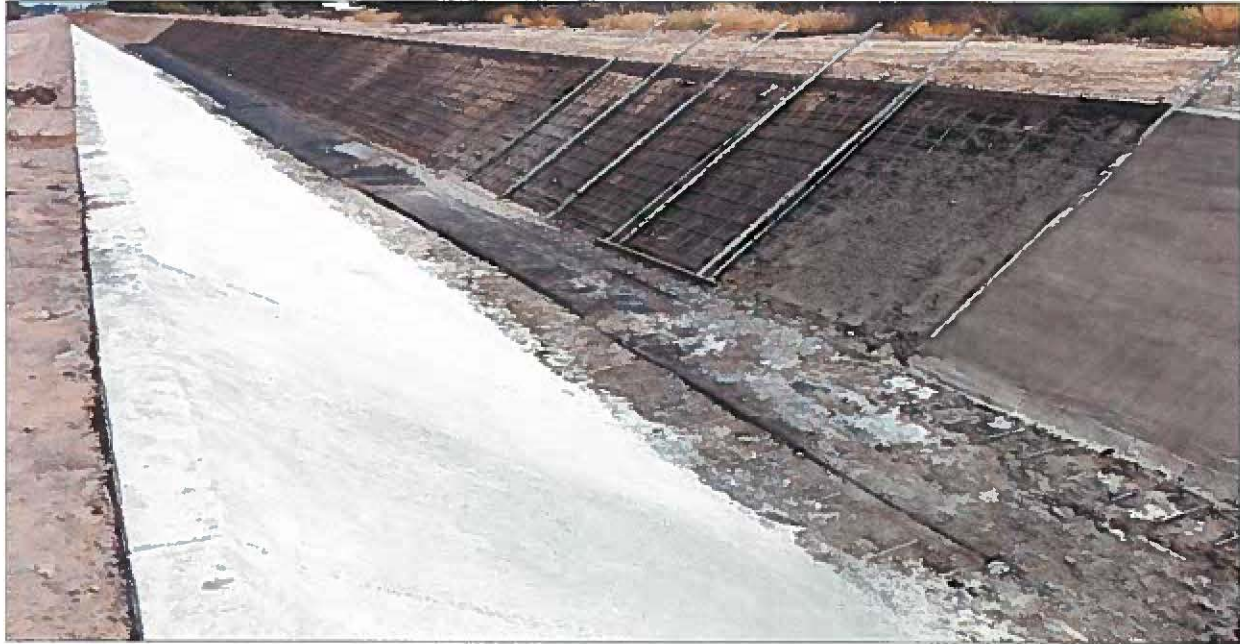
Figure 11 – Steel Panel Framework Reinforcement used at the Franklin Canal in 2019
