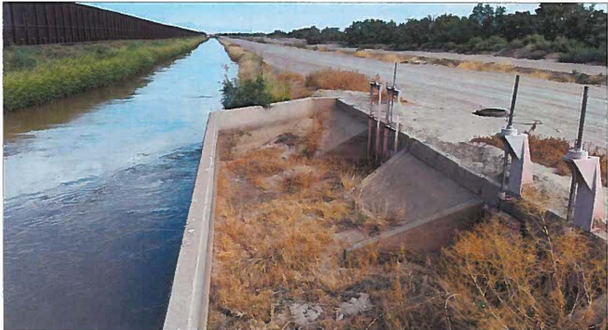
Figure 12 – Existing Release Structure at the Riverside Canal
