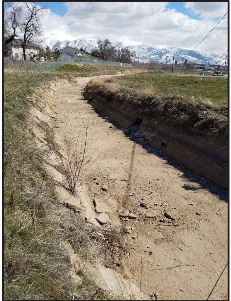
Photo 4 – DWCCC Canal Dry
