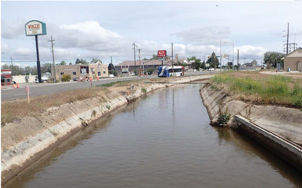
Figure 9 - Downstream measurement location. Black line indicates approximate location of measurement.
