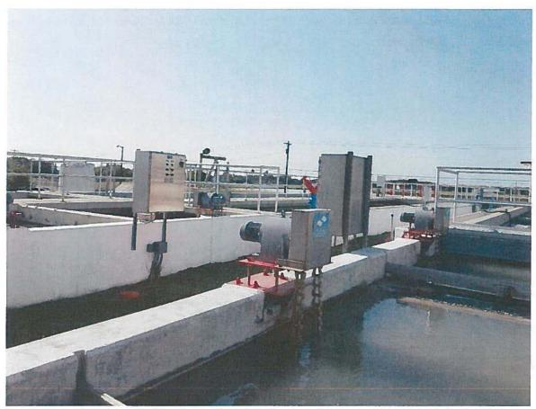
Replacement of existing TracVacs below water with pipe-less sludge mechanisms
