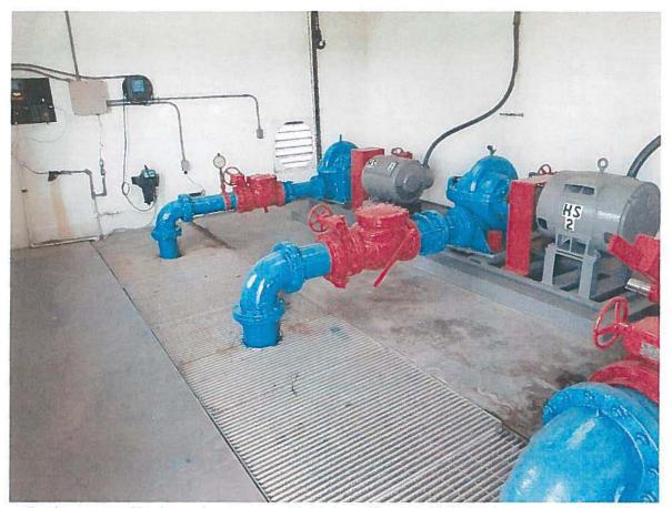
Replacement of high service pumps with higher efficiency high service pumps with VFDs
