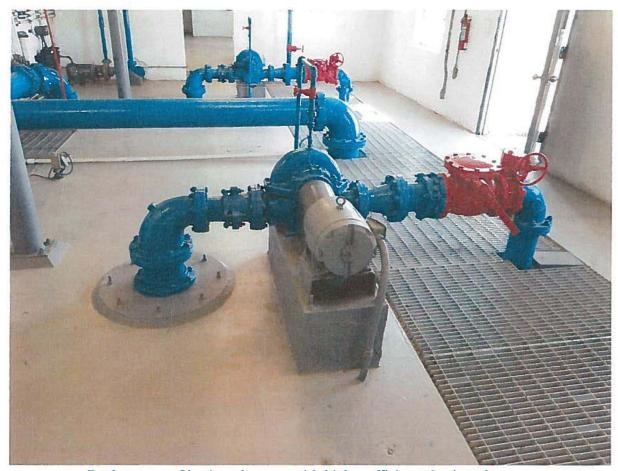
Replacement of backwash pump with higher efficiency backwash pump
