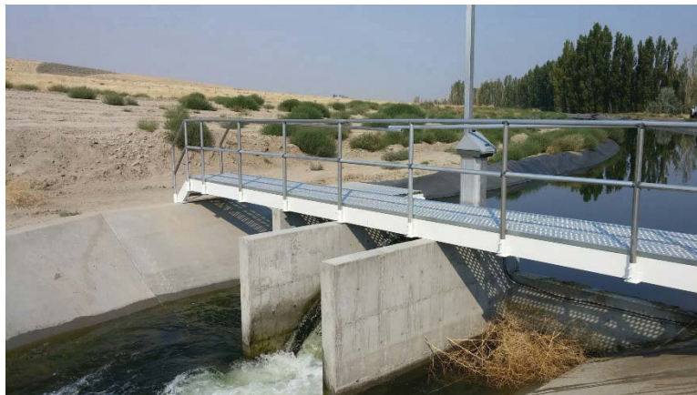
Figure 8. Handrail is installed on a walk-way plank spanning the canal.
