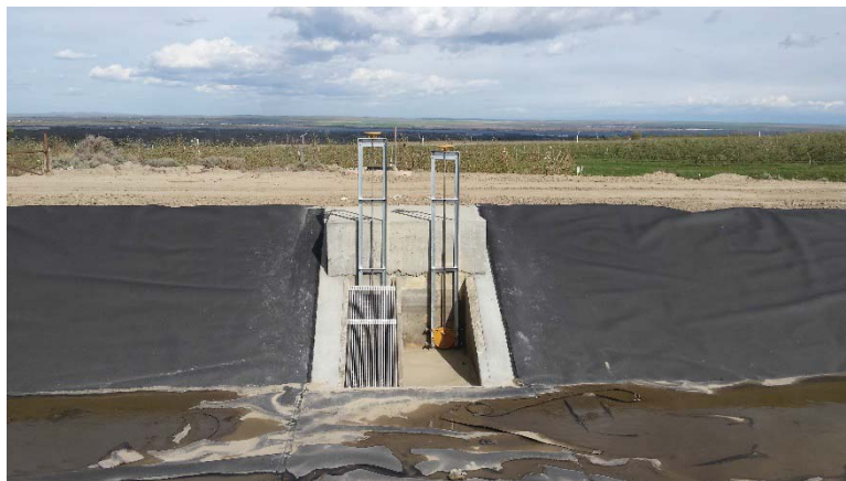
Figure 10. HDPE Welding Strip is welded to HDPE liner for full seal.
