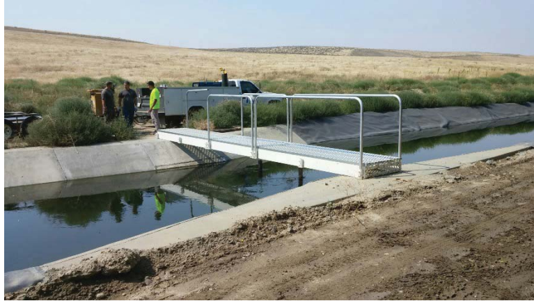
Figure 4. A typical Walk-Way Plank spanning across the canal.
