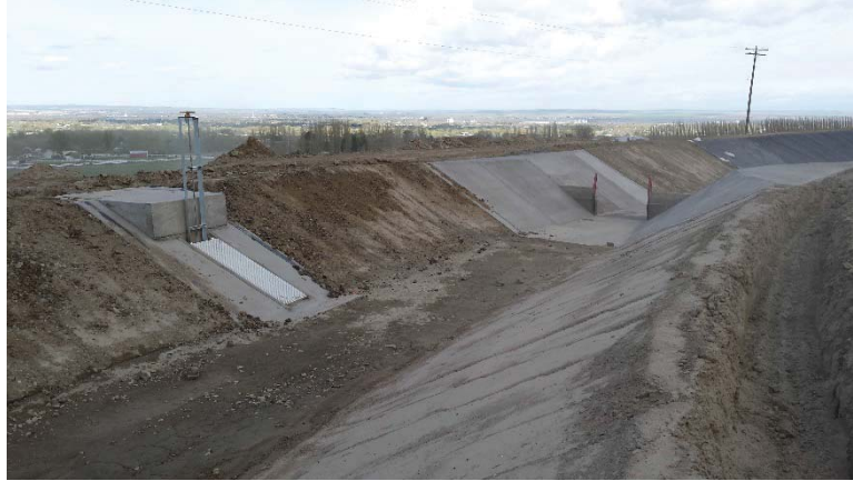
Figure 5. Modified concrete turnout (foreground) and check structure (background).
