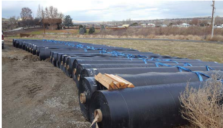
Figure 1. HDPE liner delivered to project site.
