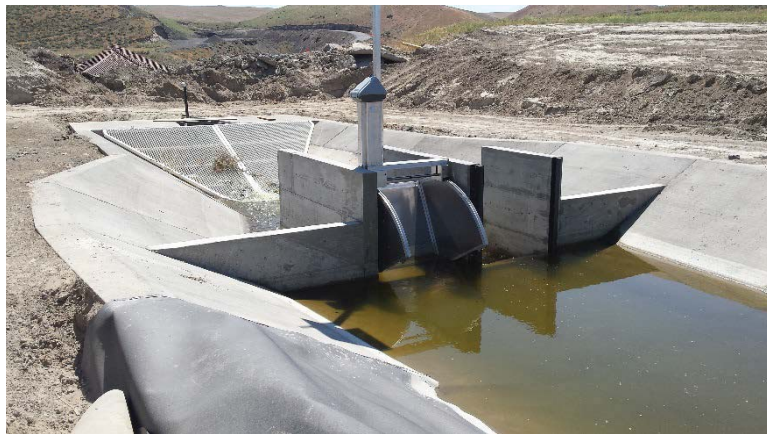
Figure 6. Modified concrete siphon entrance, with new concrete for automated flow control.
