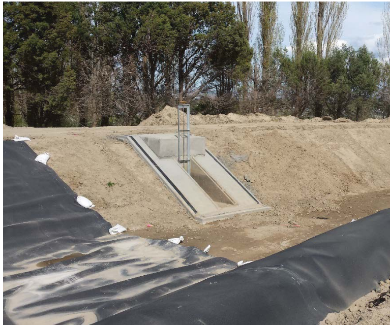
Figure 9. HDPE Welding Strip is installed on a concrete modified turnout.
