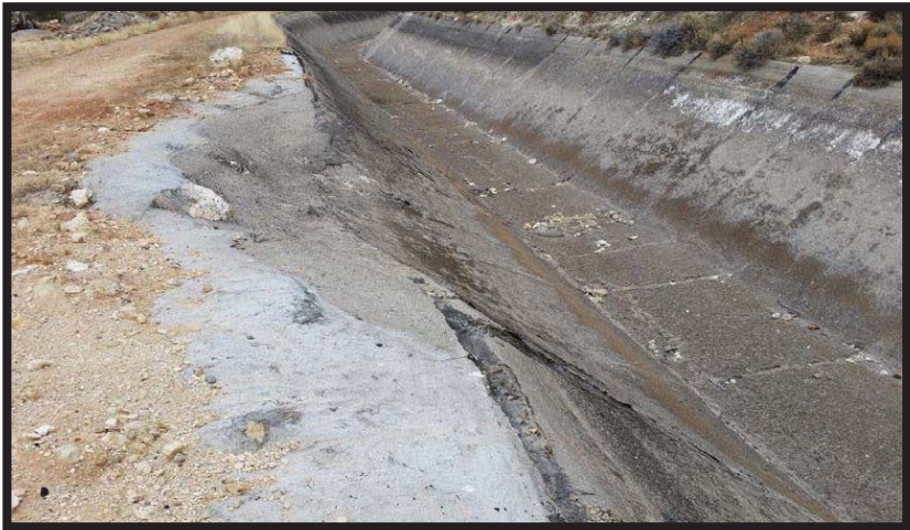
Photo 6 Canal Liner Collapse in 2011 at Station 30+92
