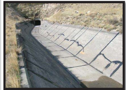
Photo 3 Grout Veneer and Asphalt Used
