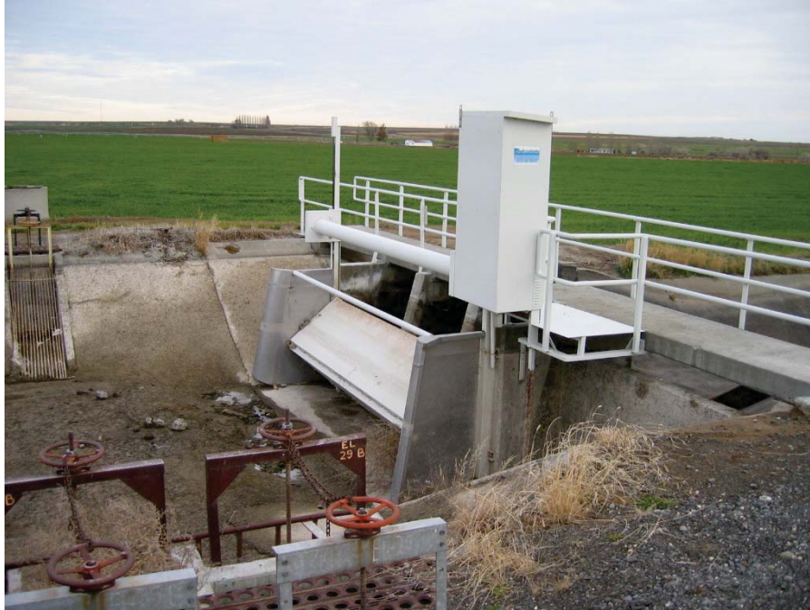
Figure 4. Example Langemann gate in existing flashboard bays
