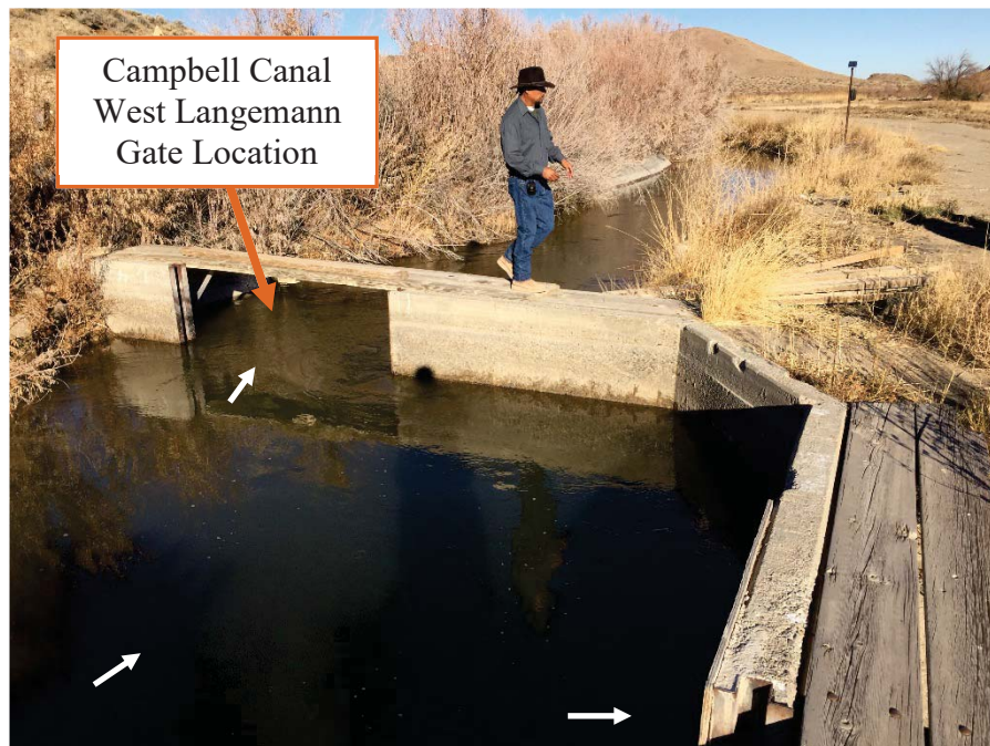
Figure 3. Campbell Canal West location of Langemann gate, Site 1
