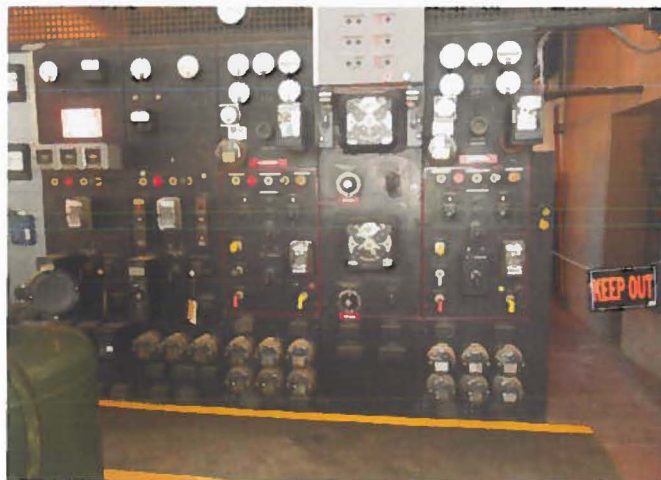
Figure 4 - GVPP Switchgear and Controls (aka Dr. Frankenstein's Lab)
