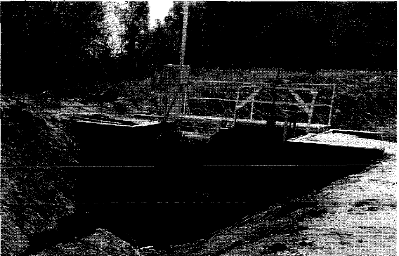
Example of proposed retrofit automated Flume Gate.
