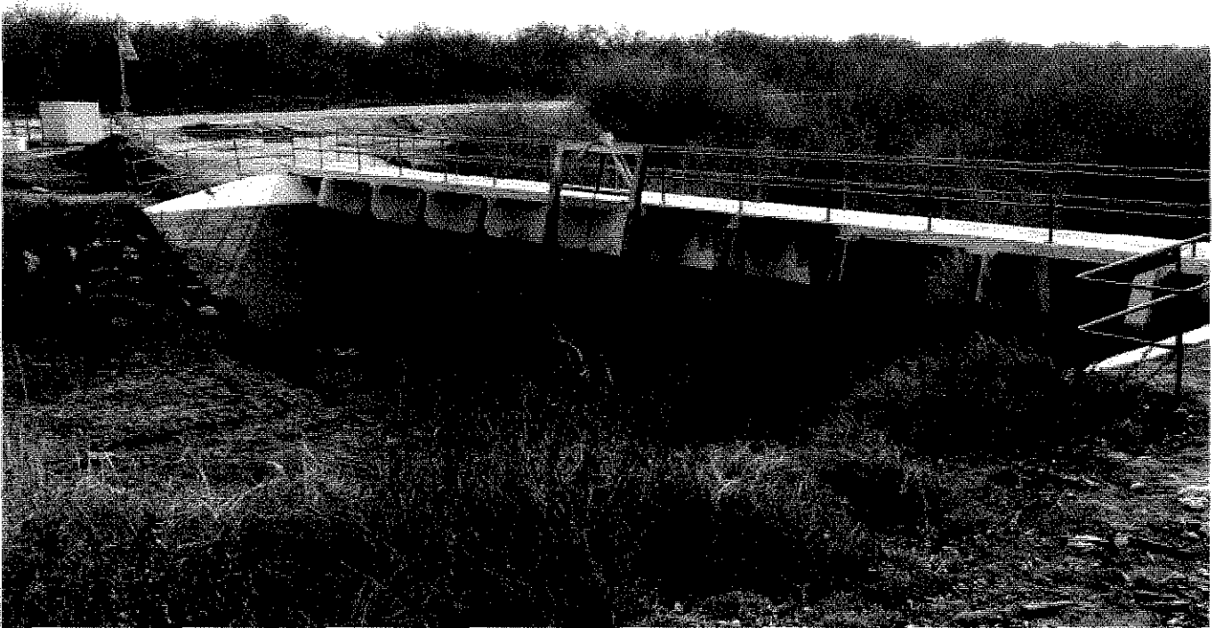
Example of proposed retrofit automated Flume Gate.
