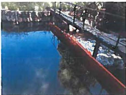
Photo 1.1-1: Stop Logs Across Sourdough Creek
