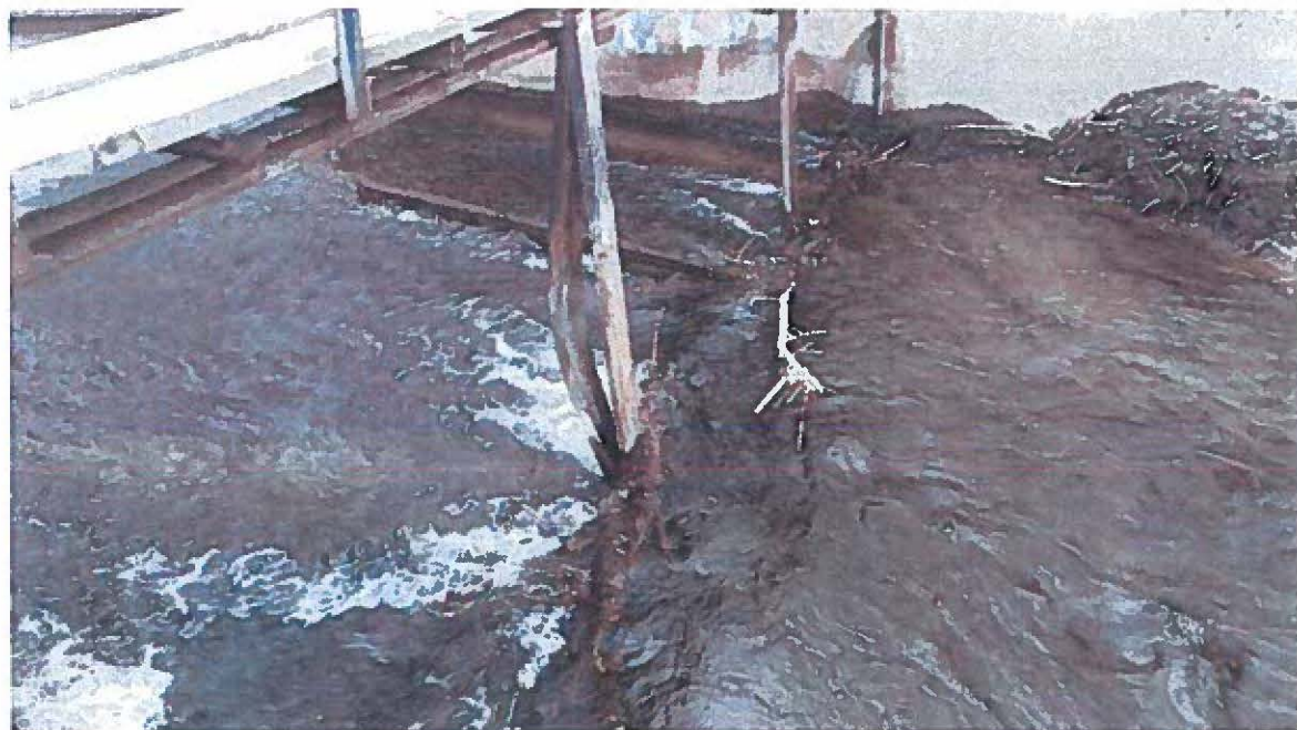
Figure 10 – Existing Diversion Dam at Sourdough (Bozeman) Creek. Notice deteriorating stop log brackets.
