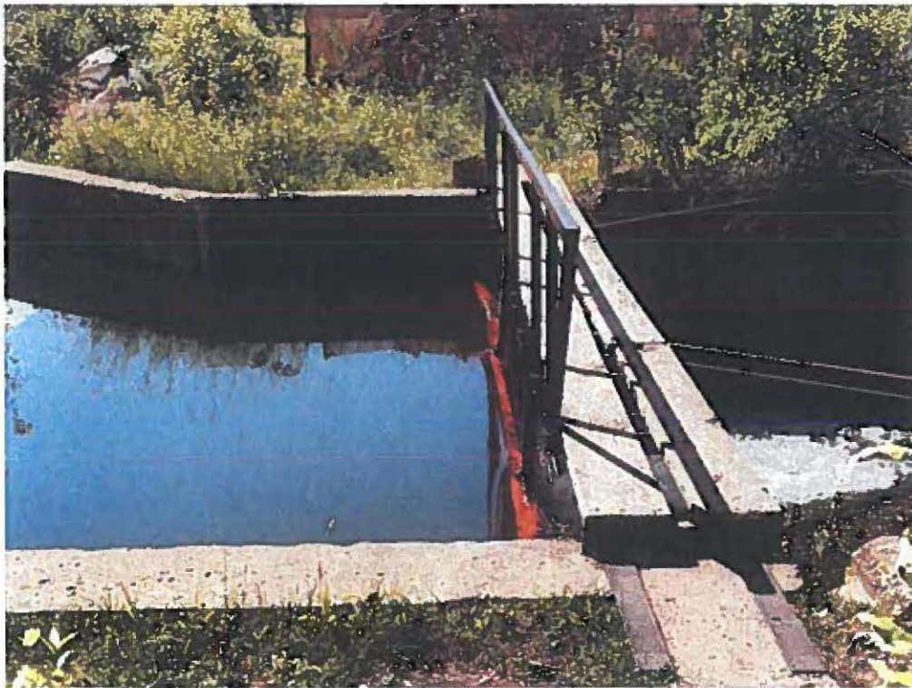
Figure 2 – Existing stop log diversion dam on Sourdough (Bozeman) Creek
