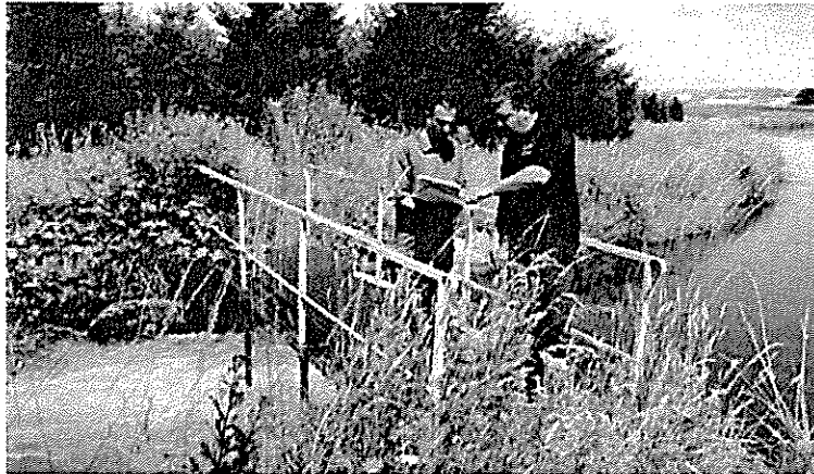
Figure 13. Looking upstream at the Main Canal. Flashboards are under the bridge, and are intended to control 50 CFS to a lateral canal. This site needs sluice gates in a well-designed cross section. The sluice gate(s) will be manual.
