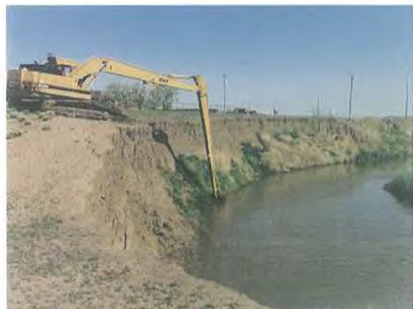
Placing barbs to control bank erosion
