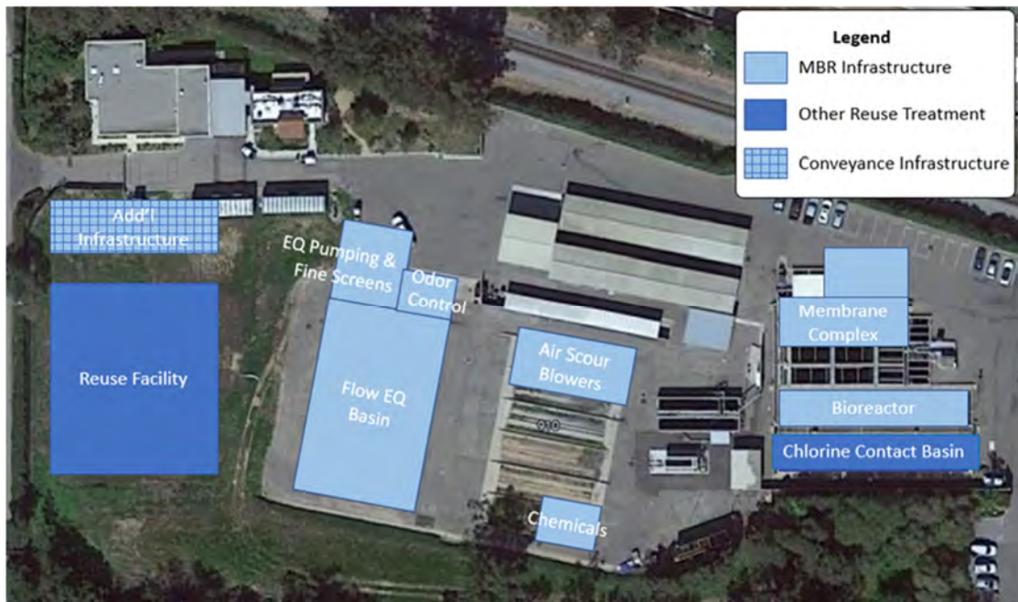
Figure 1. GAP Advanced Water Purification Facility at MSD WWTP
