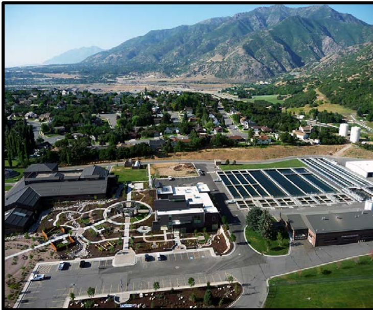
Photo 2 Weber Basin Water Treatment Facility
