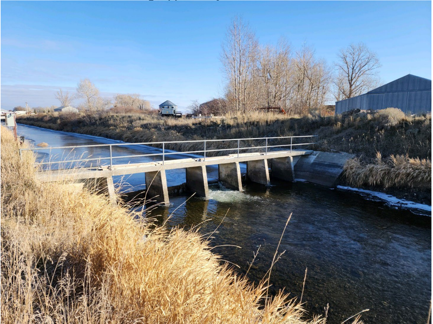
Check Structure to be automated
