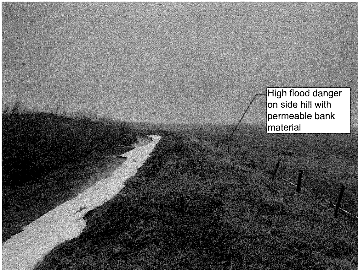
Figure 2-Marysville Canal-West End of Section to be Lined
